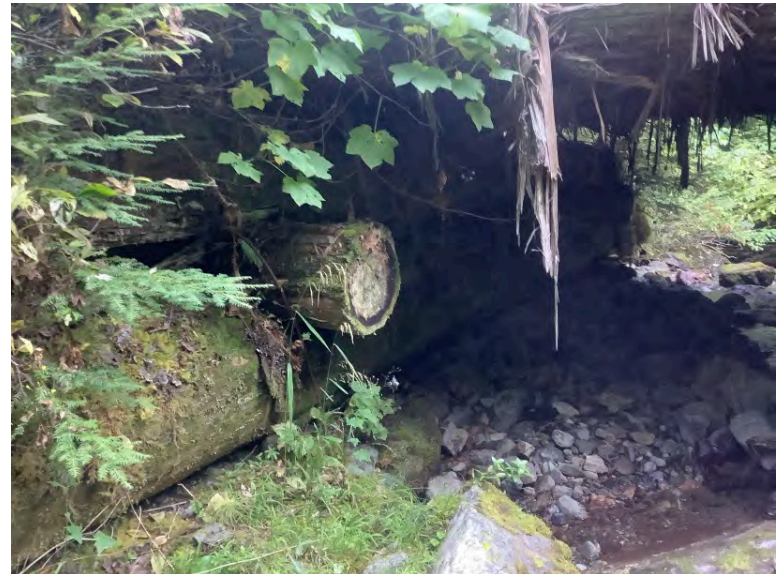
Left Bank Abutment when facing downstream
