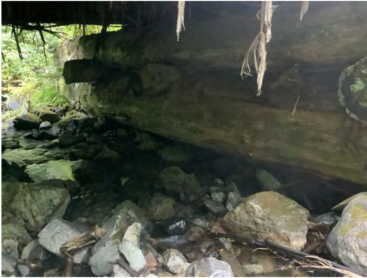
Right Bank Abutment when facing downstream
